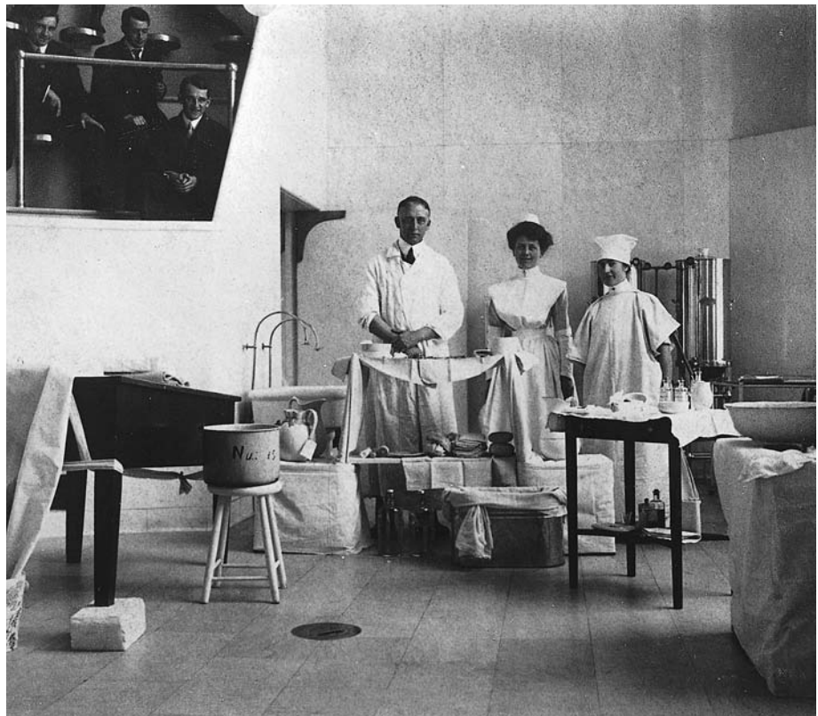
FIGURE 3-8 This early Canadian operating room—complete with a viewing gallery—was modern in its time, but it shows why many people thought that going into a hospital was risky. Make a list of things shown here that you would not expect to see in a modern operating room.
