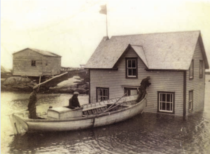
FIGURE 6–16 Resettlement continued in Newfoundland throughout the 1960s and into the 1970s. This house was towed across Inner Tickle of Newtown to its new location.
